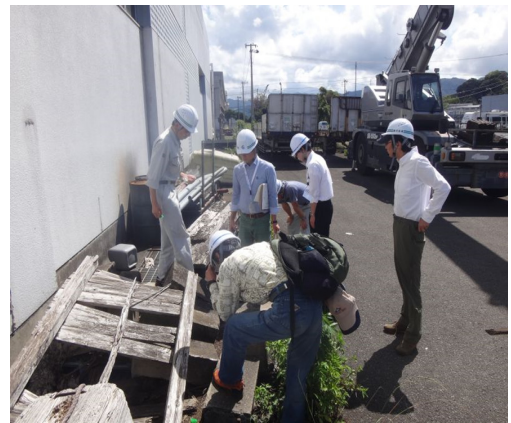
Fig. 4. Control work (Taniyama Port).
